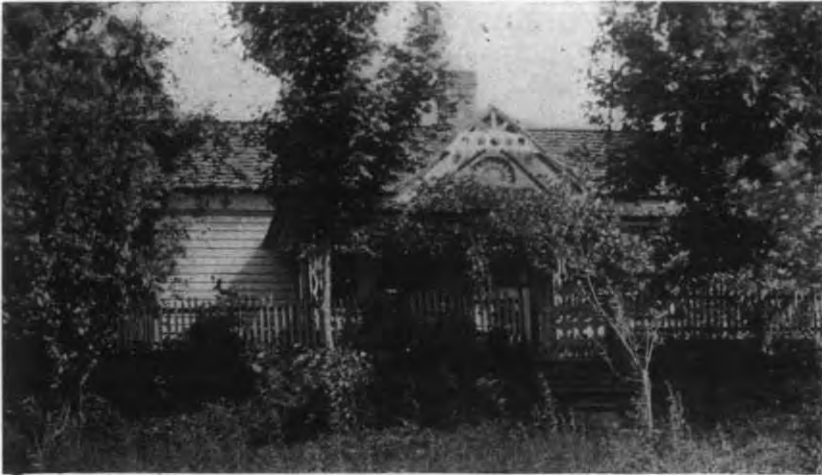
THE ORIGINAL COTTAGE WHERE THE FIRST TEACHERS LIVED
